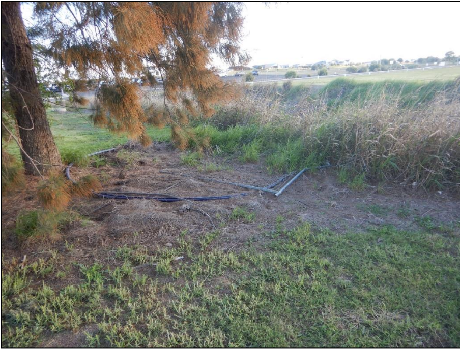
Photo B7: View of polypipe and steel temporary fence panel adjacent to drainage swale
